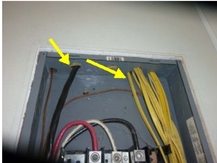
missing strain relief
