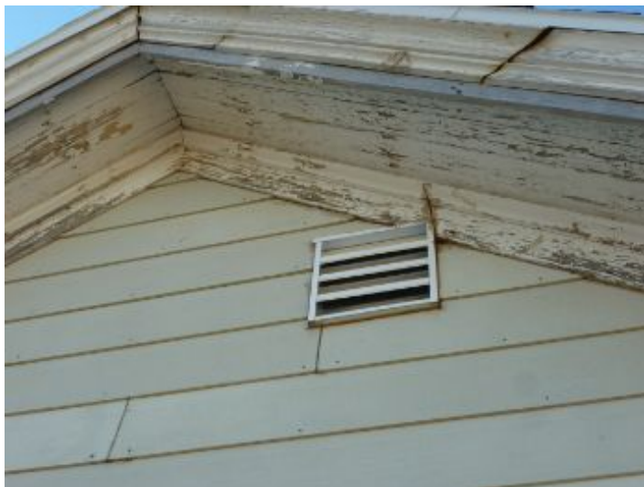
Attic Roof Ventilation
