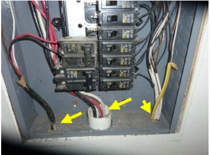
missing strain relief
