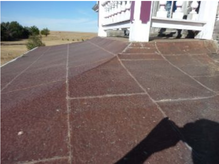
soldered tin front entry roof
