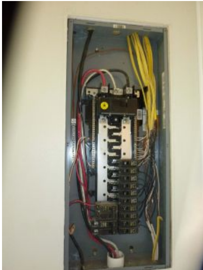
Electrical System Main Service Panel(s)
