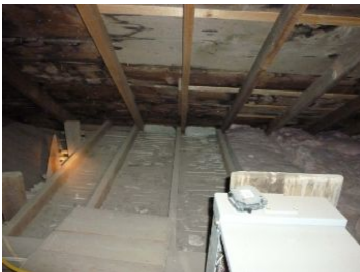
need to install missing insulation
