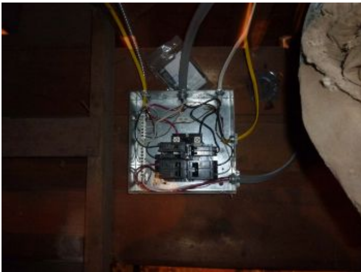
basement, needs cover installed
