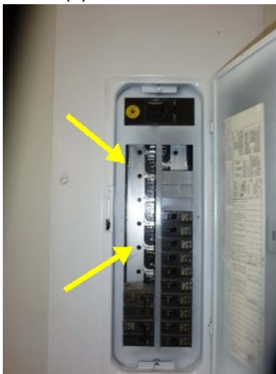
knockouts missing, safety issue
