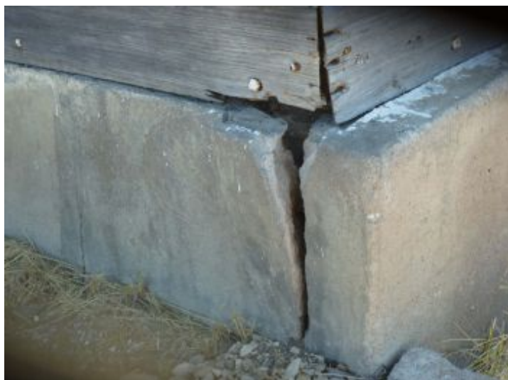
mortar crack, possible leak to interior
